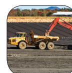
This Asheville, N.C., airport taxiway was constructed with coal ash fill.
